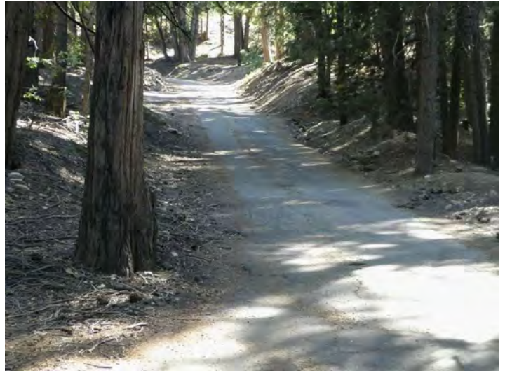
Subject street - also acts as Water District's access road to water tanks, pump house, etc.
