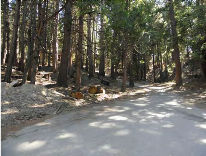
Subject street - also acts as Water District's access road to water tanks, pump house, etc.
